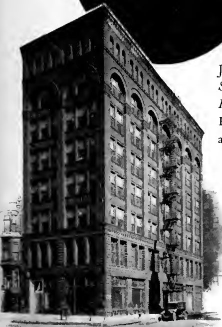
Exterior, Chicago Exchange
